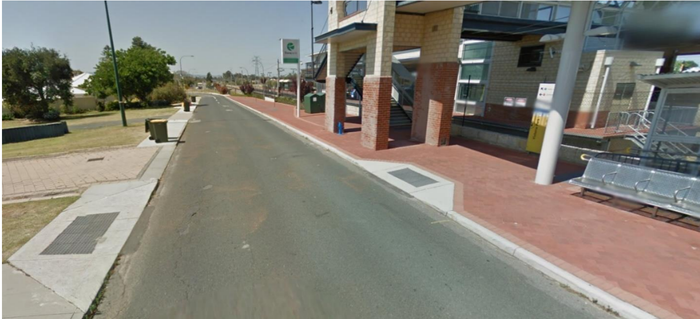
Figure 66 Rutland Avenue pedestrian crossing adjacent to Victoria Park Station entrance (source: Google Street View)
