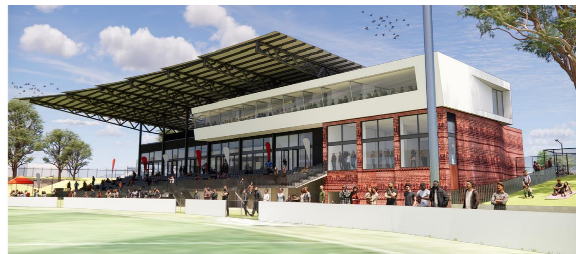
Figure 29 Lathlain Precinct Redevelopment Project – artists impression of view from oval (source: Hames Sharley, July 2023)
